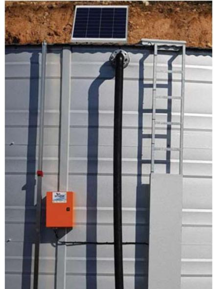
**Figure 2** A single solar panel powers the Smarta pump management system for a reservoir, dam or borehole if electricity is not available.
