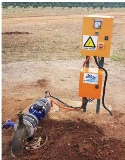
**Figure 3** This is what a Smarta system looks like when installed at a borehole. The Smarta pump management systems tells the farmer all he needs to know about his pump and pumping system, no matter where in the world he is, so that he can always operate, plan and manage his water and water resources.
