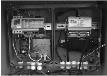
Figure 5 SMARTA Logger (Model SL001) installation example
