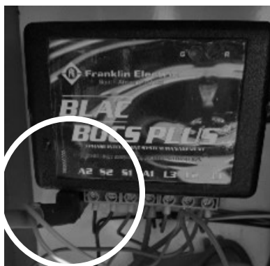
Figure 11 Blac Bocs infra-red port position
