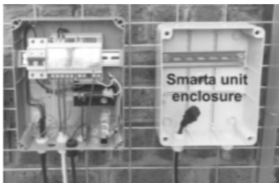
Figure 7 Mount the SMARTA Logger within one meter of the pump controller to avoid noise interference
